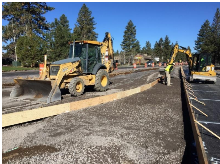
Rebuilding South Canal Blvd. starts in March 2018 and will take 13 months.
