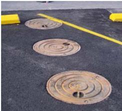
All interceptors must be cleaned periodically in order to be effective. It is time to clean your interceptor when accumulated FOG and solids exceed 25% of the total depth of the liquid or semi-annually, whichever comes first. Hydromechanical interceptors may reach that level of accumulation and have to be cleaned weekly, and gravity interceptors quarterly.
